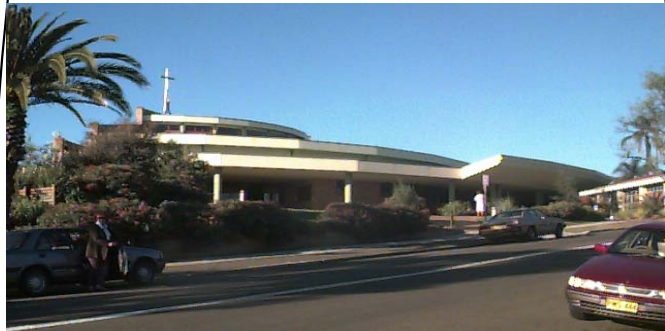
HASELER CENTRE, HILLVIEW RD, UNDERNEATH ST. KEVINS CATHOLIC CHURCH, EASTWOOD
